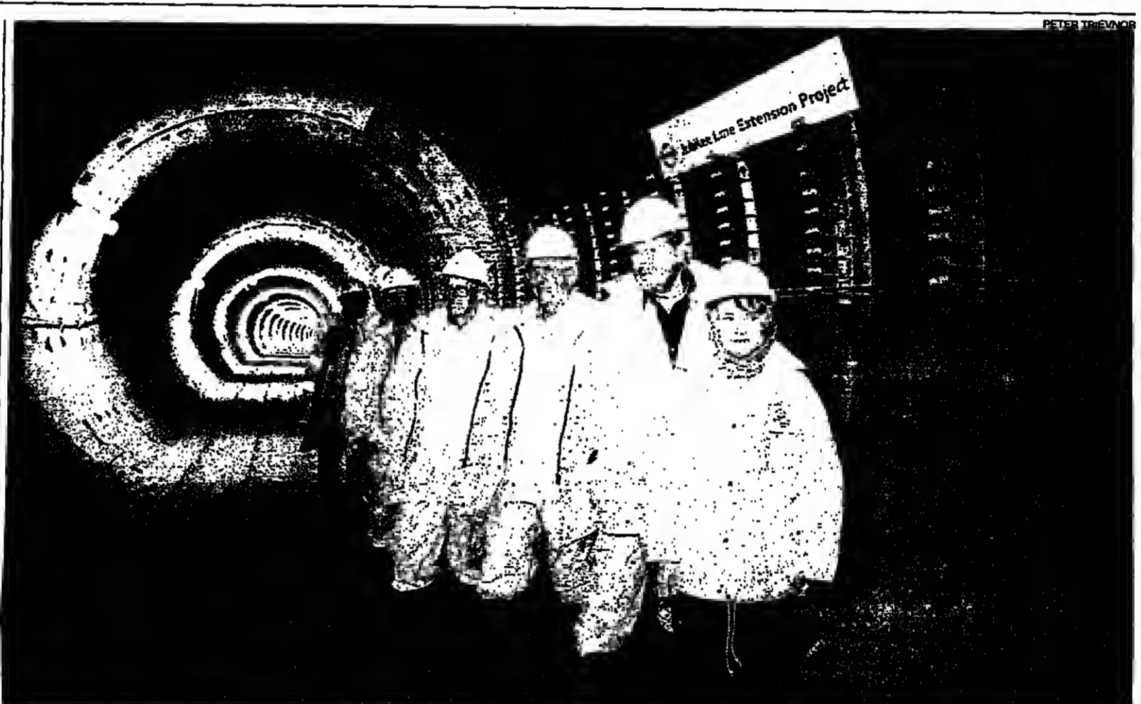
Heads of the Canary Wharf companies went for an unusual lunchtime stroll to mark the final link in the construction of the £2.5 billion Jubilee Line extension tunnel. Michael Pickard, chairman of the London Docklands Development Corp, second from right, escorted them under the Thames from Canada Water to Canary Wharf. With Mr Pickard are, from the back, Michael Smith, David Alexander, David Vaughan, Sir Peter Middleton, Sir David Walker and Colette Bowe
